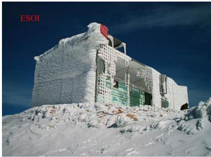
**Figure 2.** Accumulation of snow on the surfaces of the Faraday cage, which surrounds the ESOI station for lightning protection.
